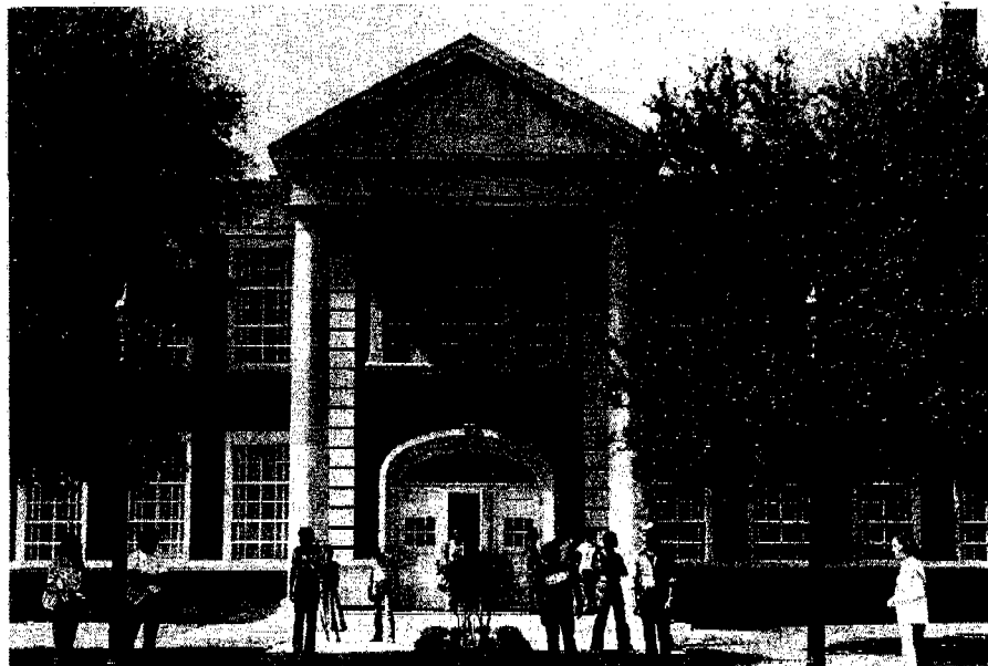
The Albritton Administration Building after renovation.
